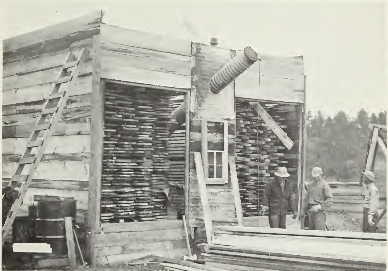
Figure 49. --Hot-air kiln being loaded.
